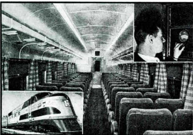
(Photo—Rock Island Lines) New streamlined "Rocket" trains, covering the mid-West at 70 m.p.h., have radio built into their light stainless-steel coaches, diners and parlor cars. The set (upper-right insert) is in diner. One speaker is shown over coach door.
