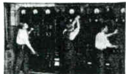
Students at COYNE operating a switchboard that controls power and light enough for a small town
