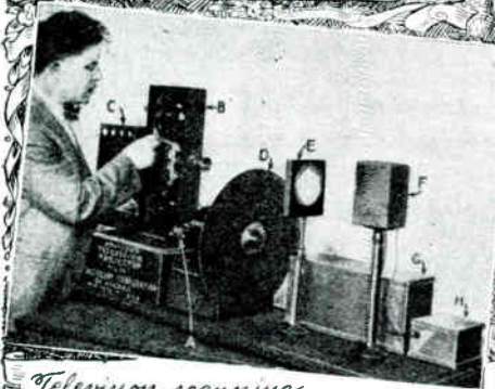
Television scanning transmitter by Insuline Corp. of America - about 1927.
