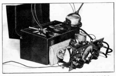
The 2-in-1 Superregenerative Receiver, with the instrument panel removed from the "card tile."
