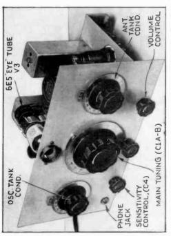
Fig. A. The neat appearance of the "Short-Wave Special." On the higher frequencies the main tuning dial affords excellent bandspread.
