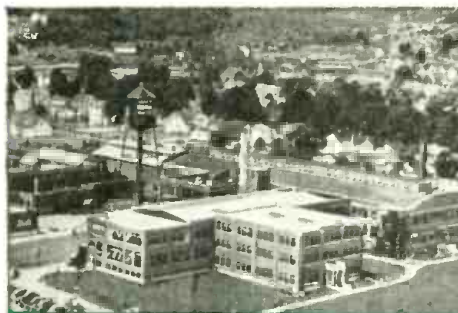
At the Emporium, Pa. Tube Plant, where pleasant surroundings help keep employees tuned to quality workmanship.
