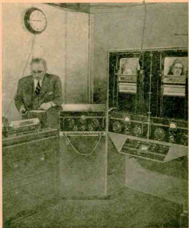
One side of transmitter console. Photo at top shows other side.
