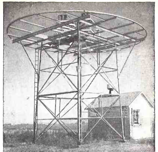
The 22-foot tower station and transmitter house for a very-high-frequency radio range.
