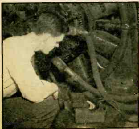
Fig. 2.—DON'T put them here! Strong fields from the cables may ruin the calibration.
