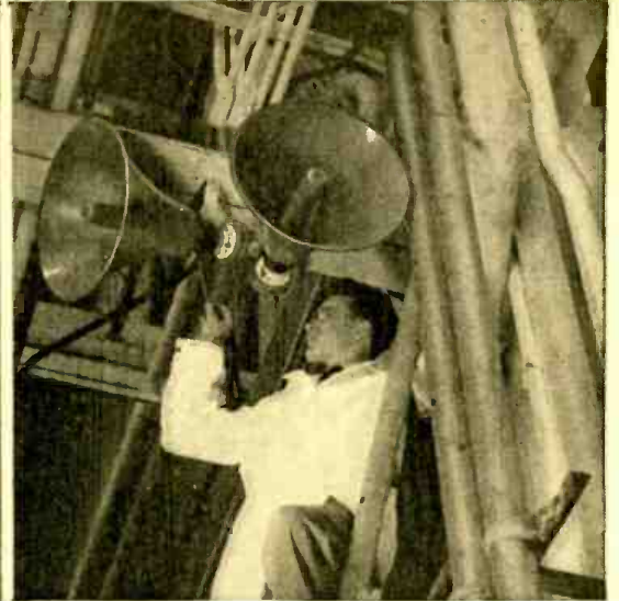
Above—Two of the Atlas Sound DR-42 Dynamic Reflex Projectors installed in the Pratt & Whitney Aircraft engine assembly building. There are 3 speakers in the cluster, one being hidden by the column. Left—Three 75-watt power stages mounted in rack, together with two-position mixer. Switching permits progressive paging by groups of seven speakers to each power stage. The whole system is controlled from one point, where a "grip-to-talk" microphone is used.
