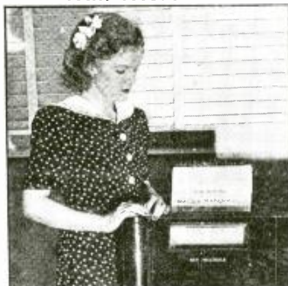
Facsimile transmission and reception is a feature of the RCA exhibit at the N.Y. World's Fair, and this pretty watches the special facsy edition of the N. Y. Evening Post come in. Material, sent to Fair from N.Y.C. by messenger, is transmitted from a facsy pick-up in the exhibit.
