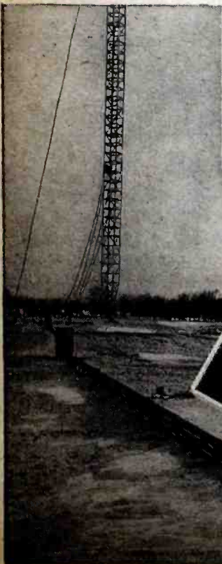
WHAS , 650-ft. vertical radiator fed by a 50-kw. W.E. transmitter. Note the nitrogen-filled coaxial transmission lines.
