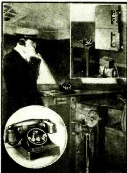
Fig. K. Ten frequencies are available in the 50-watt transmitter and receiver designed by Western Electric for coastal vessels. Unit shown is remote control. Insert, transmitter, which user's voice automatically turns on. Circle, phone rings on calls.
