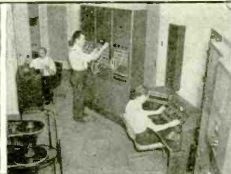
6 The Central control room, where the material piped to the pylons is monitored and distributed. Engineers here can direct the sound all over the grounds, or confine it to the radius of a single pylon, at will.
