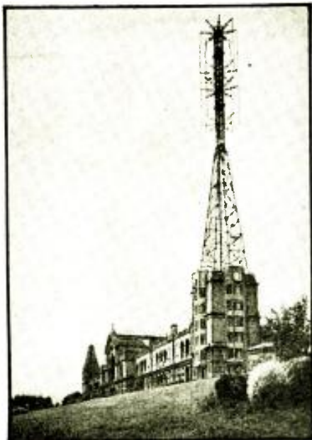
The tapering tower for the 2 transmitter aeriels.
