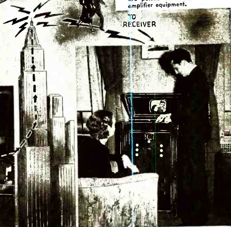
FIFTH—RECEPTION. The images and accompanying sounds are picked up in special cathode-ray television receivers which are synchronized with the scanning of the transmitter. Images 7 1/2 x 10 ins. can be obtained. (Receiver details appear on page 74 of August 1936 RADIO-CRAFT.)
