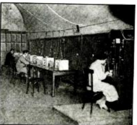
A section of the French reception center with switch-board to the Postmaster's office.
