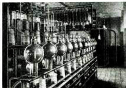
Rectifier panel of the Budapest broadcast station.
