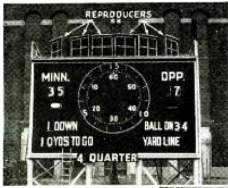
Six Wright-DeCoster reproducers in a large horn furnished adequate coverage for 65,000 people at Michigan U's stadium.
