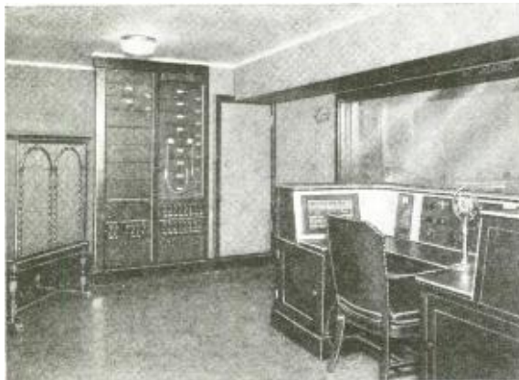
Two typical views of network equipment in a national chain; the studio monitoring and output control boards.
