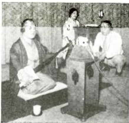
This photo shows an interesting experiment in broadcasting conducted recently by a Japanese radio network, in which several blind musicians broadcast simultaneously from different locations. Telephone lines were used to cue the programs.
