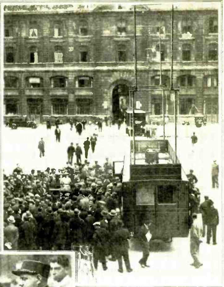
T HE two photos, above and to the left, show a new installation just completed in Paris, for providing radio aid to the Prefecture of Police. The transmitting car, with its large aerial structure is shown above, while one of the patrol cars equipped with receiving apparatus appears at the left.
