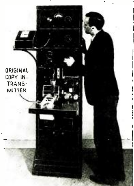
Fig. B Pictures being sent on the special transmitter.
