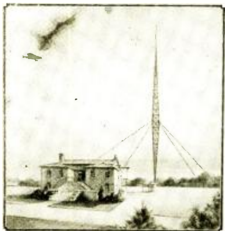
Fig. A The mast antenna and the transmitter house.
