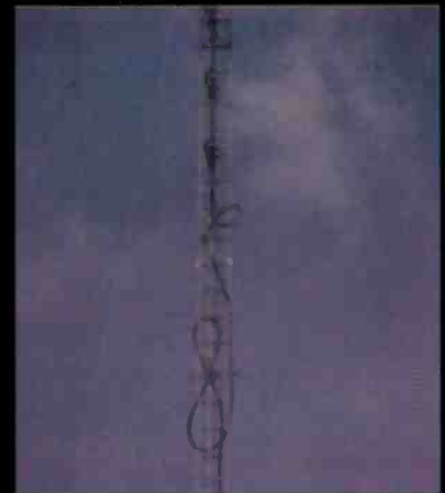
An extreme case of poorly dressed and secured transmission line
