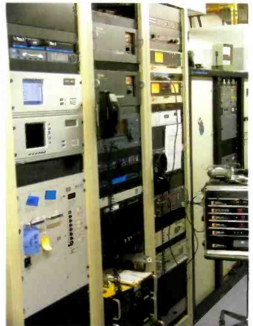
Entercom's KQBZ/100.7 HD Rig, The misc racks are to the left and behind the Continental 816R FM Tx. The monitor array to the right is used by all stations for mod level set up etc.
