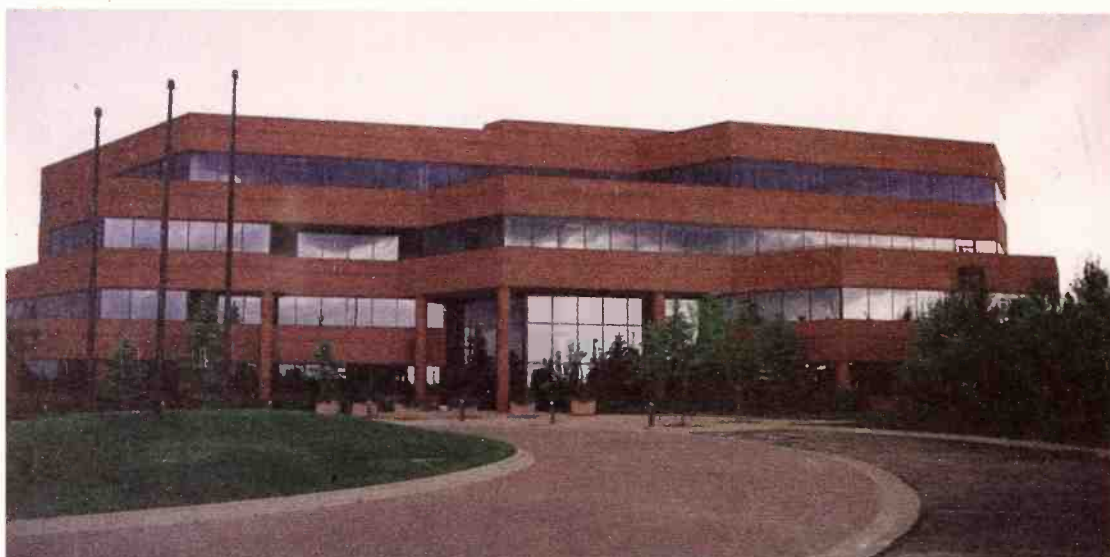
Clear Channel's new Denver HQ: 85,000 sq. ft., four floors and a basement host all facets of seven radio stations. Of the whole building, only a small area will be leased out on the first floor. That area will serve as reserve space for future expansion needs. Engineering takes the basement.
