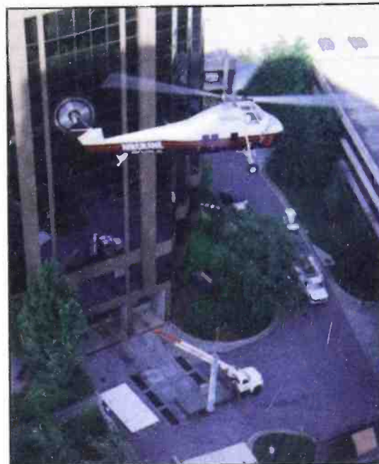
A helicopter raises the new monopole antenna mount for WAMJ-FM
