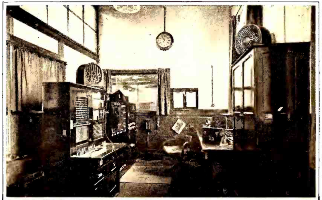
CONTROL ROOM OF 3 LO, MELBOURNE
