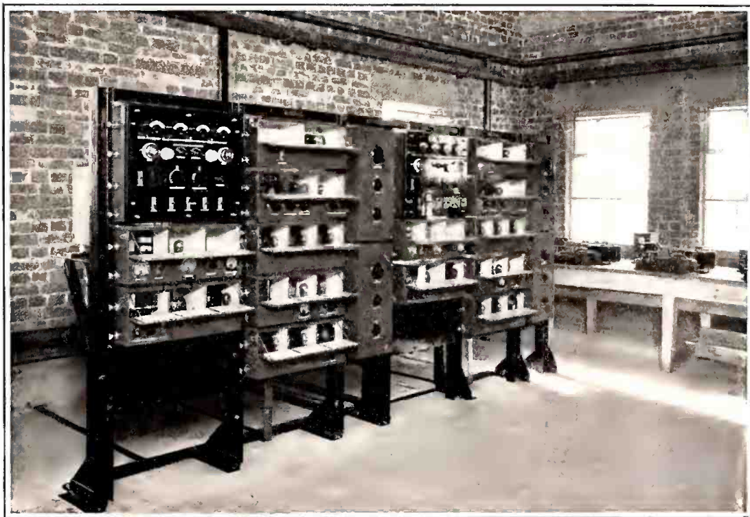
RECEIVING EQUIPMENT AT THE BRIDGEWATER STATION
