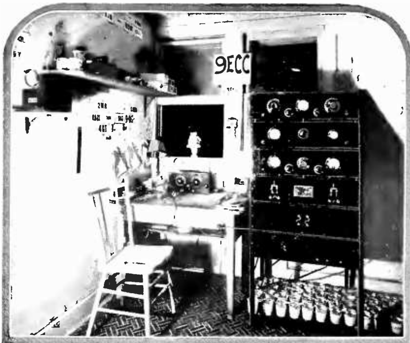
STATION 9ECC AT MINNEAPOLIS Note the chemical rectifier on the floor and the businesslike transmitter arrangement
