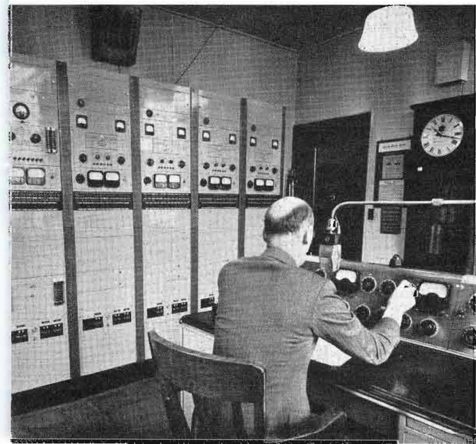
Operator at the master control console of transmitters at Bound Brook.
