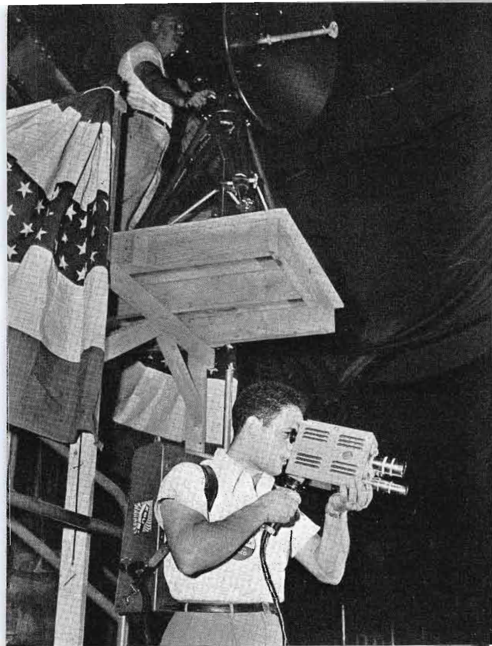
Portable walkie-lookie unit is dwarfed by a huge parabolic receiving unit used to pick up microwave signals from walkie-talkies on the auditorium floor.
