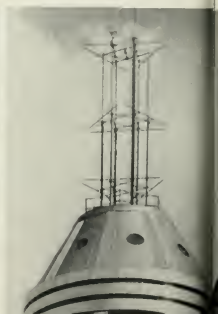
1936—AN ARRANGEMENT OF POLES AND RODS SUPPORTED THE THREE TRIANGULAR ANTENNAS OF THE SECOND STRUCTURE TO BE BUILT.
