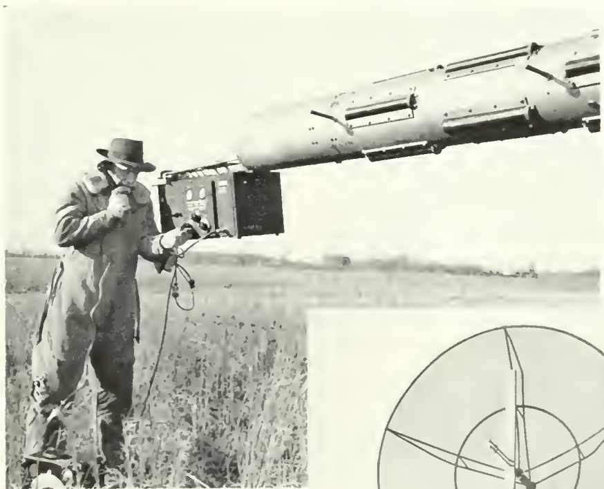
ENGINEER TUNES SLOT-TYPE ANTENNA BEFORE IT IS LIFTED TO TOP OF 210-FOOT TOWER OF BRIDGEPORT STATION.
