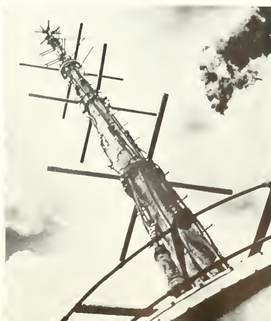
1946—THE PRESENT 61-FOOT SUPER- TURNSTILE ANTENNA WAS ERECTED WHEN NBC COMMENCED TELEVISION TRANSMISSIONS ON CHANNEL 4.
