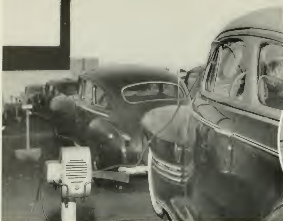
LOUDSPEAKERS SUSPENDED ON PEDESTALS BETWEEN ROWS OF CARS ARE DRAWN THROUGH A WINDOW AND ATTACHED AT THE MOST CONVENIENT PLACE FOR THE OCCUPANTS.
