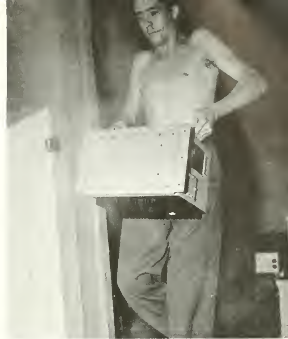
SHIPBOARD INTERCOMMUNICATION UNIT BEING BROUGHT FROM "TORTURE CHAMBER'S" WEATHER ROOM, WHERE IT OPERATED IN 140-DEGREE HEAT.
