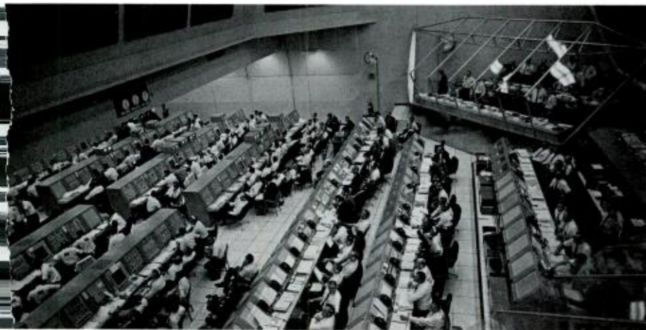
The firing room at Cape Kennedy contains display, monitoring, and control equipment. Every critical component of the rocket was automatically checked out by RCA computers during the launch sequence.
