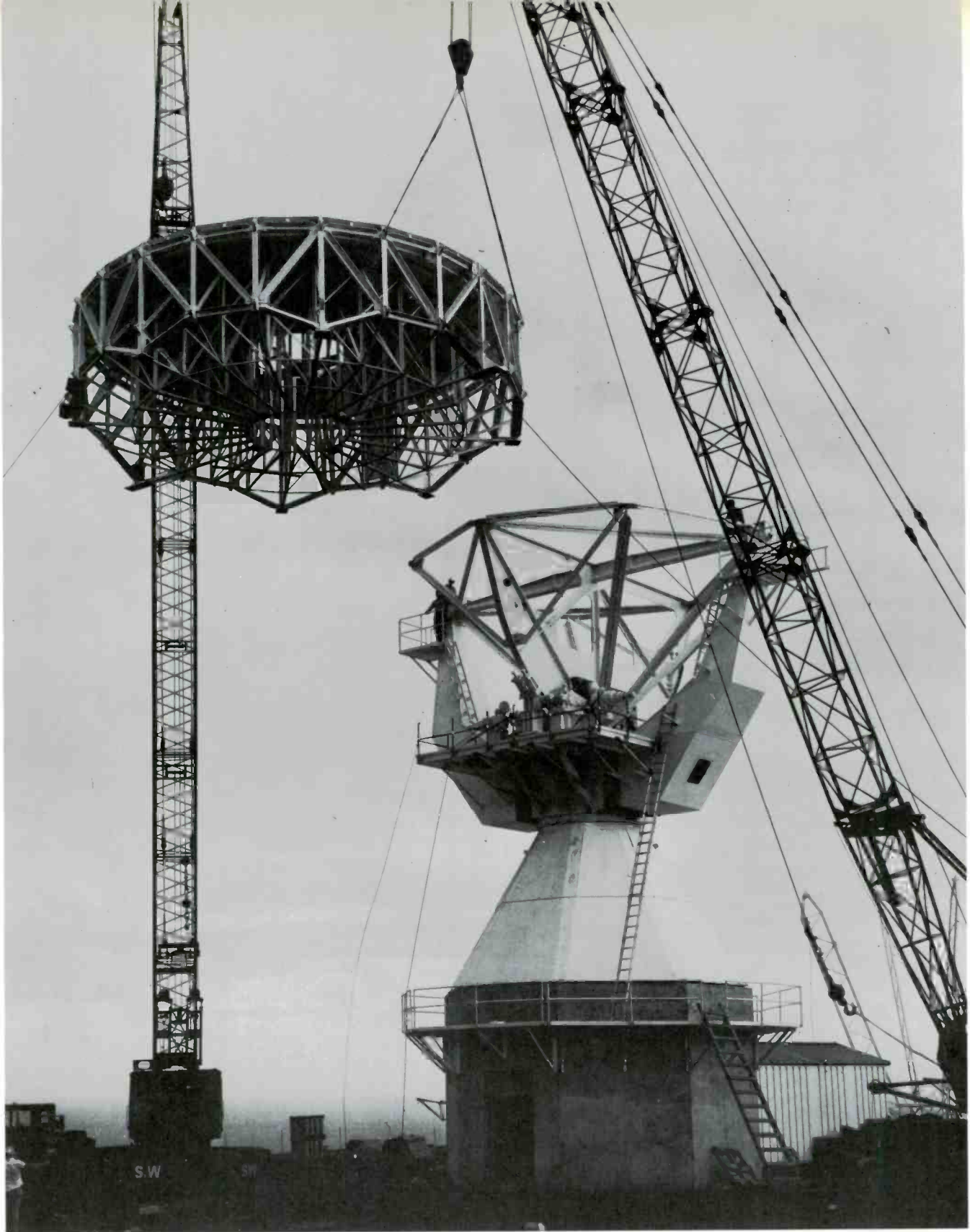
An antenna reflector is assembled at Paumalu, Hawaii. When complete, the station will be a key link in a satellite communications system serving the Pacific area.
