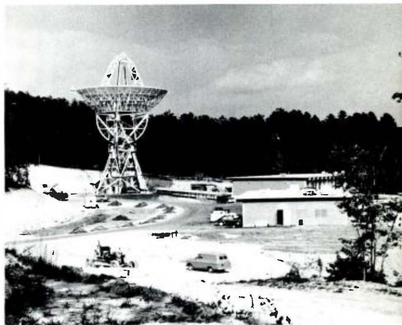
Ready for data from space. The North Carolina Data Acquisition Facility can handle the most complex experiments.
