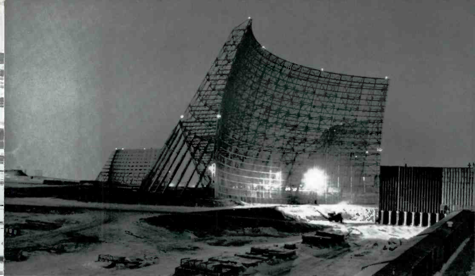
Four of these giant antenna reflectors at the Thule, Greenland, BMEWS site provide data on missile speed, trajectory and impact area.
