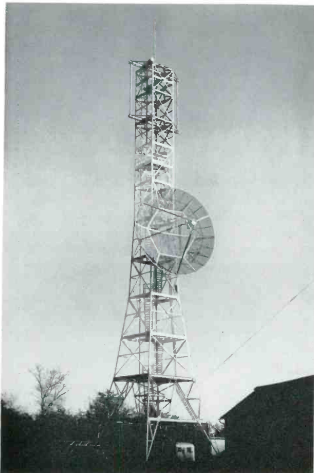
An RCA Laboratories experimental tropospheric scatter antenna at Riverhead, L.I., receiving station.
