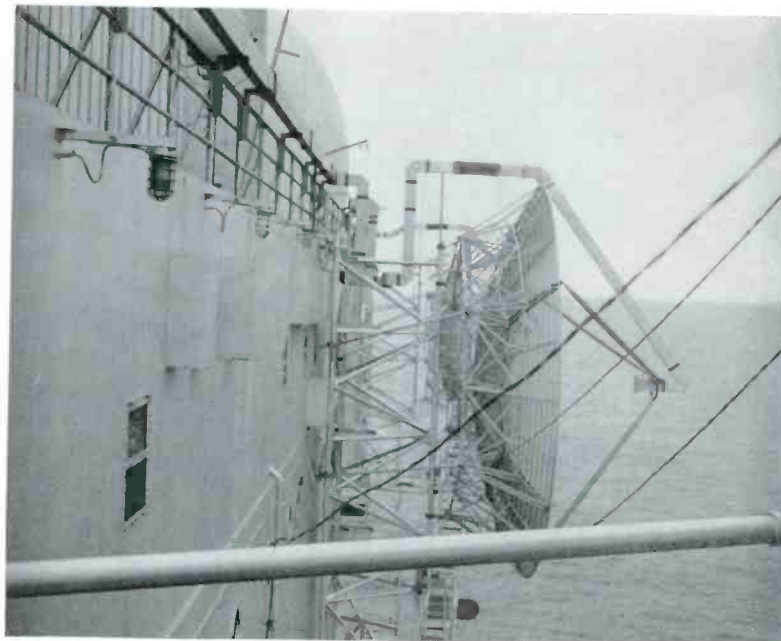
Tropospheric scatter antennas mounted on the side of a new Texas Tower radar installation in the Arctic.
