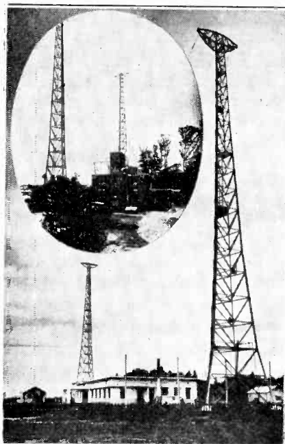
In the oval is shown a view of the old 1 kilowatt station used by JOAK. It is now used as a studio only, situated on Mt. Atago, (Atago-Yama), in Tokyo. The large picture shows the newer 10 kilowatt JOAK building and towers, located at Shingo, north of Tokio. These photographs were taken by Hidewo Kikutani, formerly Chief Engineer of the Japanese shortwave experimental station J1AA. (Courtesy of Mrs. Dora Newcomb).
