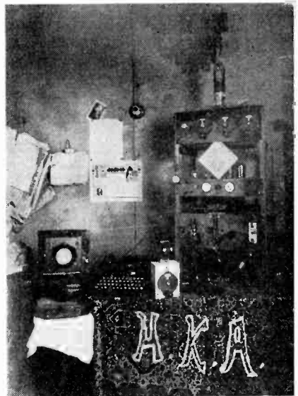
Little HKA is a good sample of the tiny transmitters which provided our shortwave fare back in 1931. The 50-watt tube had to be put on top as there was not room for it within the transmitter proper. The home-made microphone is shown to the left. Sr. Jesus Amortequi was the owner of this station, located in Barranquilla, and served as Engineer and Announcer as well. The English announcer was Ed Ilera, who can still be heard at times announcing in English from certain Barranquilla stations, particularly HJ1ABG.
