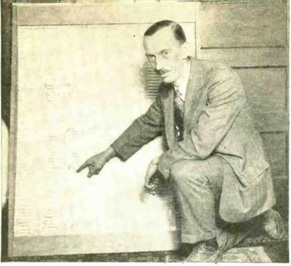
A NEW IDEA IN LOUDSPEAKER CONSTRUCTION Instead of the familiar magnetic coil construction of the ordinary loudspeaker, this unique reproducer unit, the patented invention of Collin Kyle, of San José, Cal., employs electrostatic attraction and repulsion as its operating principle. The complete absence of mechanical parts prevents it from getting out of adjustment, and the large vibrating surface makes for distortionless reproduction.
