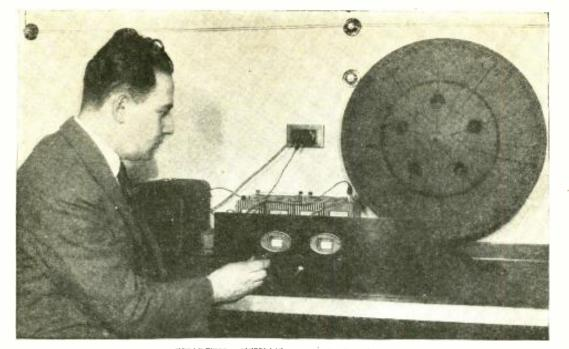
QUALITY RESULTS WITH A CRYSTAL. After the preliminary adjustment of the auxiliary controls, the operation of the New Home receiver is accomplished with the two tuning drums and the volume control knob.
