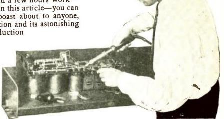
A JOB THAT THE BEGINNER CAN COMPLETE The soldering of the connections on the Counterfonic becomes an astonishingly easy job, by reason of the extreme simplicity of the wiring. Nearly all the wires are run under the sub-panel.
