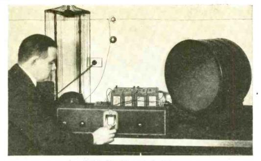
THE VICTOREEN IN OPERATION The Victoreen is shown here operating with a loop antenna; however, one of the features of the new receiver is its adaptability to operation with other kinds of antennas, such as the light socket and outdoor types.
