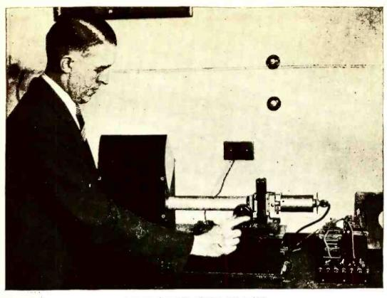
MAKING A HUM SHOW ITS PATH By means of the oscillograph, shown in the picture above, oscillating currents are made to trace, on a screen, luminous paths showing their wave form. The engineer is shown testing the output of a power-pack with this delicate instrument in the POPULAR RADIO Laboratory.
