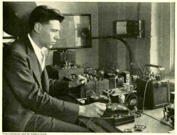
HOW VOLTAGE-REGULATION CURVES ARE RUN ON AUTOMATIC FILAMENT ADJUSTERS FIGURE 1: The set-up that was used to make the curves that are given in Figure 3. The cir-
