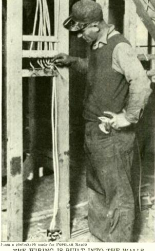
THE WIRING IS BUILT INTO THE WALLS The wiring for the outlet box for the switches may be done before the plaster has been put on the wall, as shown here, or it may be threaded through the wall partitions by a competent electrician.
