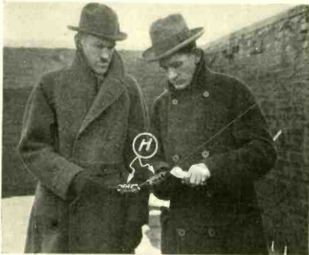
HOW THE INSULATORS ARE ATTACHED FIGURE 5: The two insulators, shown at H, should be connected in series between the antenna wire proper and the hoisting wire.
