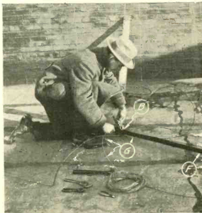
ATTACHING THE GUY WIRES TO THE TOP PIECE OF THE MAST
