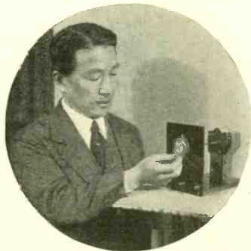
Even the absent-minded professor could not forget to tune in on a radio program with this invention of Ushichiro Tokumi, attached to his set. It will turn a radio set on or off at any time you wish, by closing an electric circuit when the clock reaches the hour at which the indicator is set.
