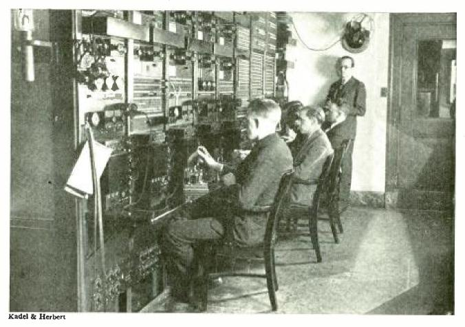
HOW BROADCAST STATIONS ARE LINKED TOGETHER BY WIRE Here is a long-distance control board for the telephone lines that are used to connect a number of widely separated broadcasting stations, so that they may all transmit the same broadcast program.
