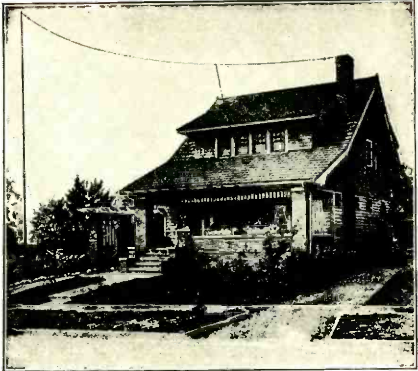
40 Ft. Mast in Yard
