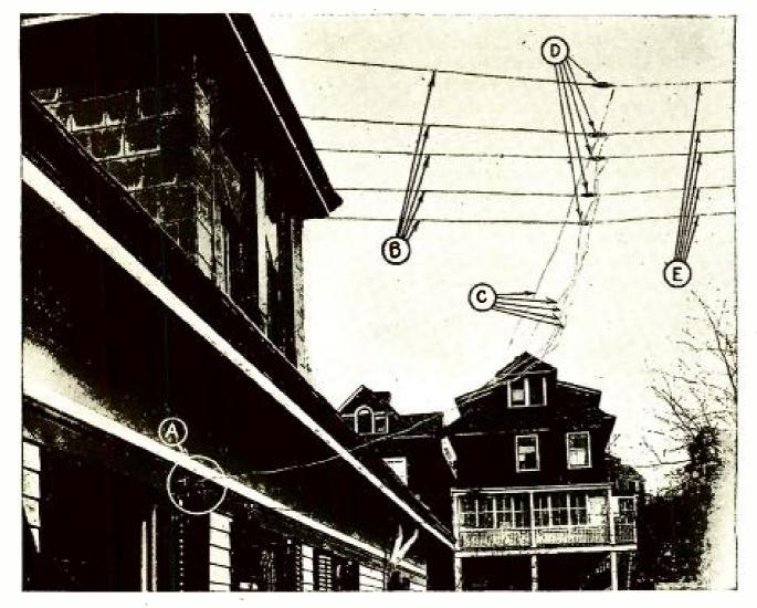
THE LEAD-IN END OF A WELL-CONSTRUCTED ANTENNA A is the lighthing switch; B the supporting wires; C the lead-in wires which are joined together to form a common lead-in; D the insulators and E the antenna wires that run to another set of insulators and supporting wires or ropes. It will be noted that the antenna is placed out from the tin roof of the house a distance of at least fifteen feet; this is done by lengthening the wires or ropes B.
