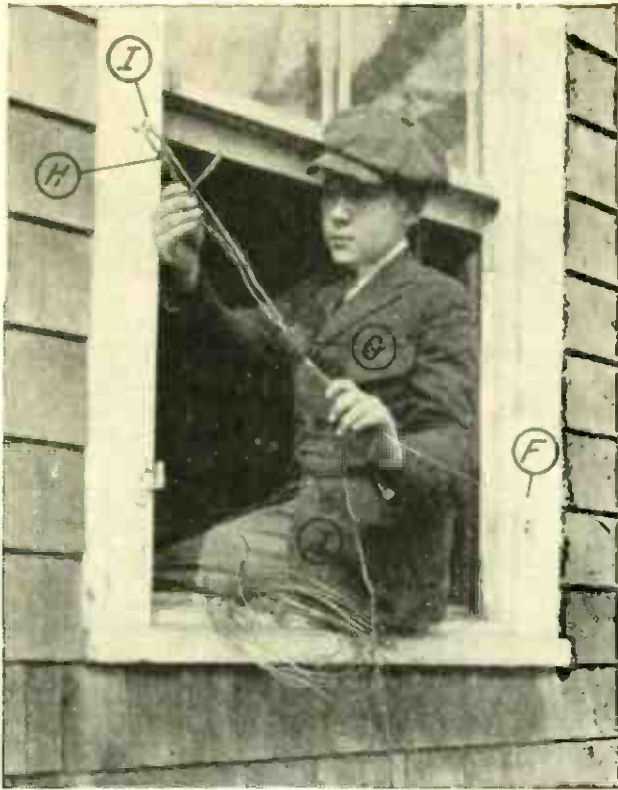
I Fastening the insulated lead in wire to the antenna wire. F is the antenna wire, G is the insulator; H is a piece of rope, I a screw eye and J the lead in wire.
