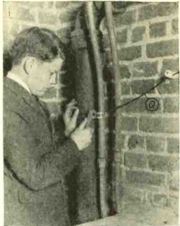
IV How the ground lead is attached to the water pipe by means of a ground clamp. Q is the ground wire.
