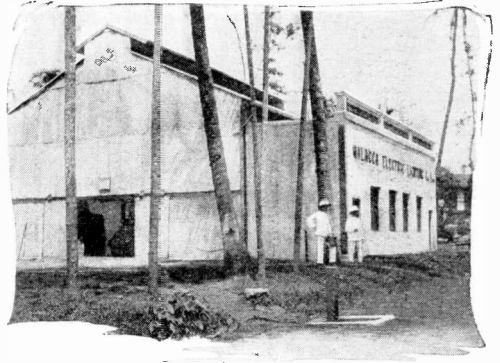
Electric Plant of Malacca
