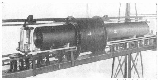
GENERAL FEATURES OF THE LEVITATED SYSTEM: (I) ALUMINUM BED-PLATE; (2) IRON BODY OF CAR;
