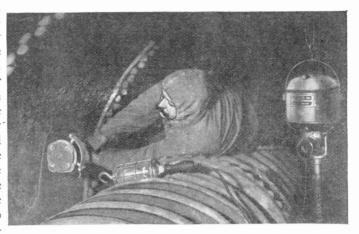
REMOVING BOILER SCALE
