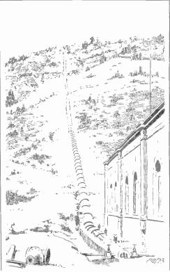
A MOUNTAIN STREAM IS CONDUCTED THROUGH A 30 INCH PIPE TO THE HYDRO-ELECTRIC PLANT
