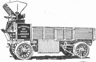
Gutterson  $\mathcal{R}$  Gould of Lawrence, Mass., are using this  $3\frac{1}{2}$ -ton Electric Truck for healing junk. It actually saves 24% over horse haulage; gives greater elasticity of operation.
