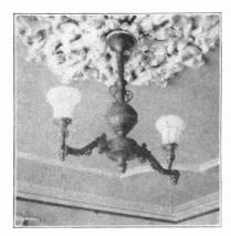
GAS FIXTURE CONVERTED TO ELECTRIC
