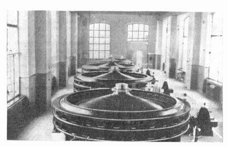
DYNAMOS IN A SWISS POWER PLANT, DRIVEN BY WATER TURBINES
