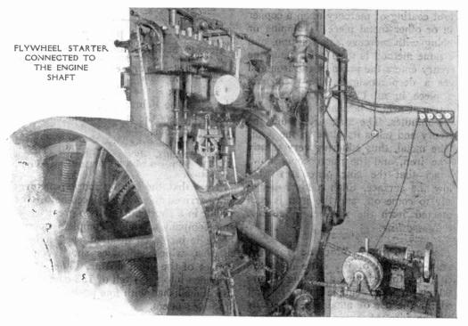
stroke of the piston before the charge can be exploded and start the engine to running of itself. This operation is most familiar in the laborious cranking of an automobile engine. In stationary engines, too large to crank by hand, the work is often done by a separate compressed air equipment, which is expensive and, if it fails to accomplish its purpose,
