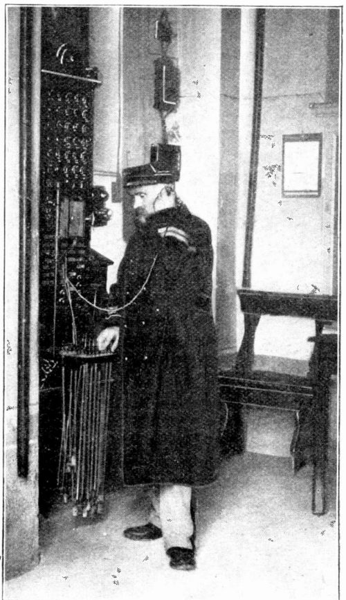
TELEPHONE SWITCHBOARD IN THE VATICAN, IN CHARGE OF A UNIFORMED ATTENDANT
