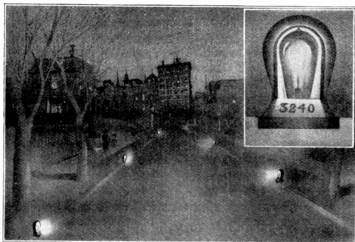
CURB STREET LIGHTS AND HOUSE NUMBERS
