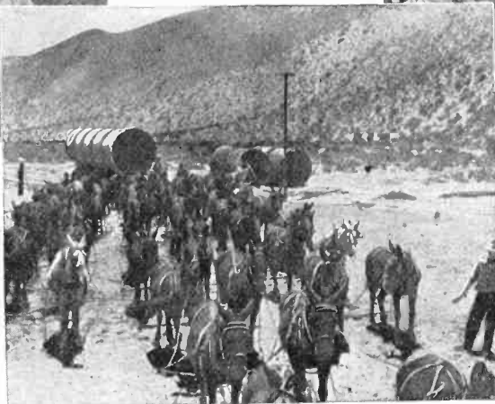
52-Mule Team Hauling Steel Sections for the Saugus Siphon.
