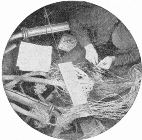
CABLE SPLICER AT WORK
